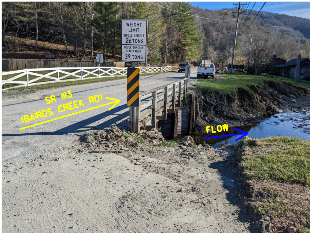
PHOTO #2: VIEW FACING SOUTHEAST.
