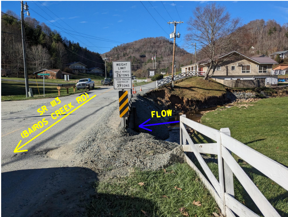
PHOTO #1: VIEW FACING NORTHWEST.
